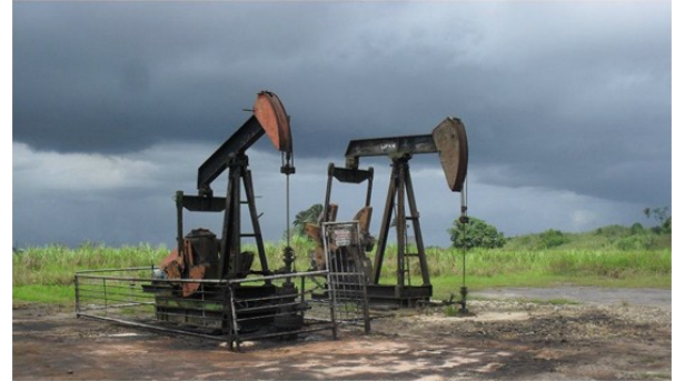
Pumping Jacks in the Barrackpore Oilfield, Southern Basin Trinidad
